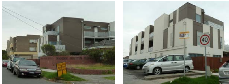
Recent three storey development on Virginia Street
