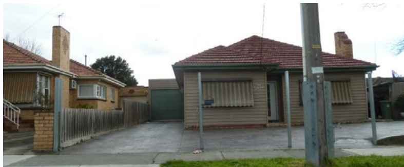
Single storey development along Merton Street
