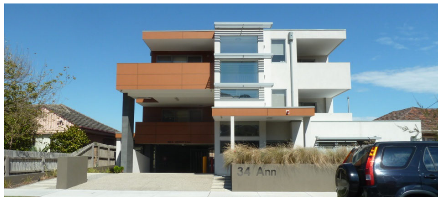
Examples of recent three storey development in Precinct 2
