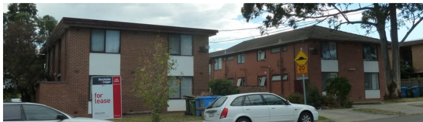
Existing development along Potter Street
