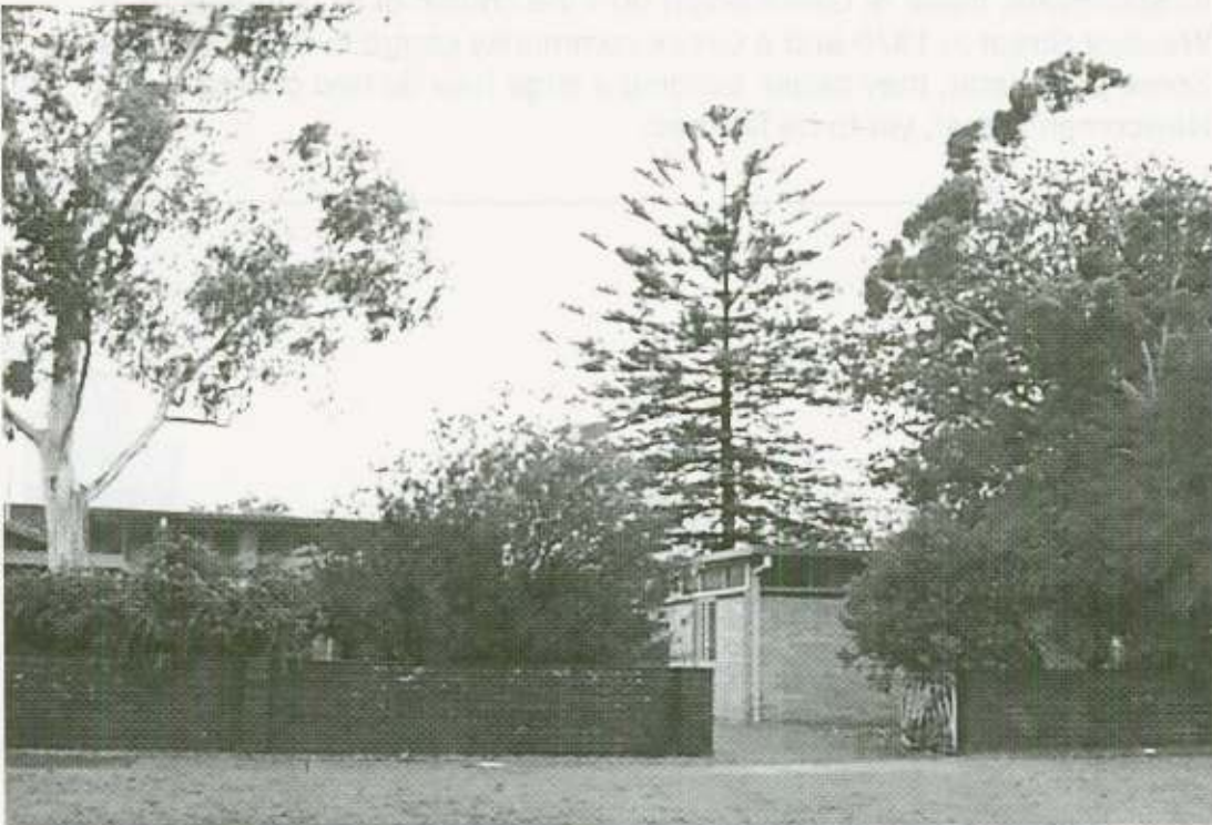
Figure 5 Pickett Street Lutheran Church, Dandenong
