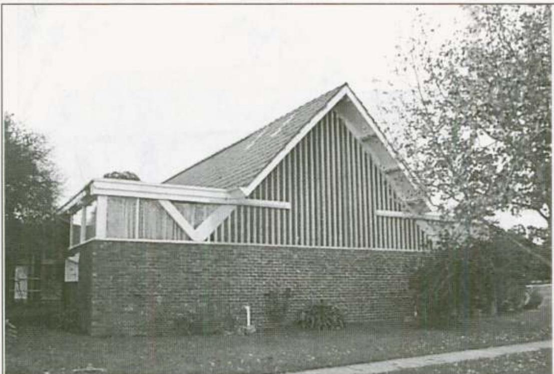
Figure 30: Dandenong Presbyterian Church, designed by Chancellor & Patrick
