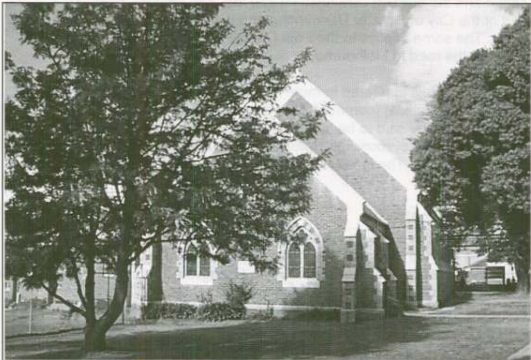
Figure 28: Dandenong Uniting Church (rear)
