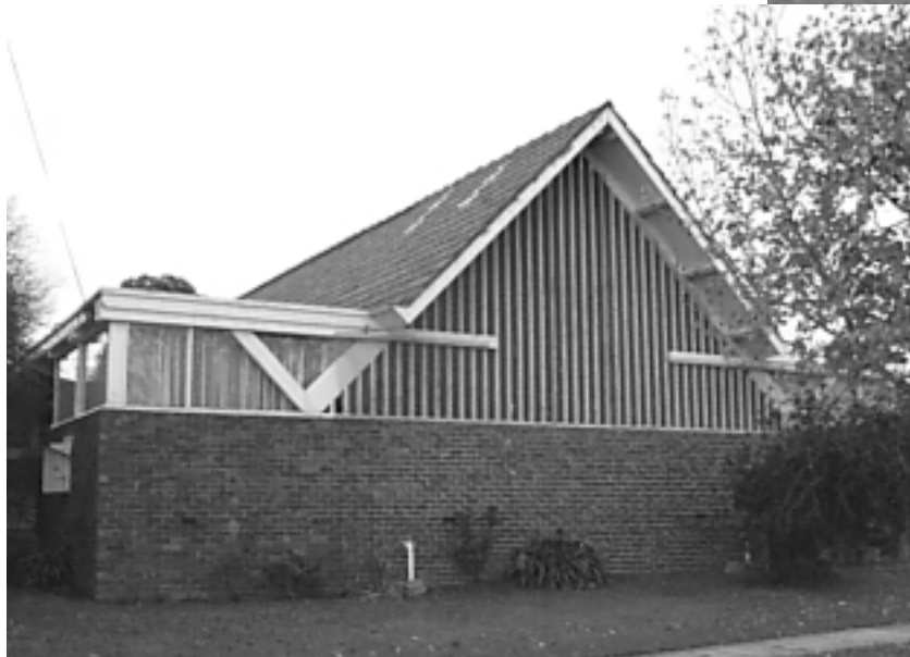
Figure 30. Dandenong Presbyterian Church, designed by Chancellor & Patrick
