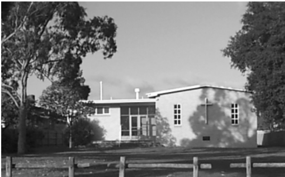
Figure 5. Pickett Street Lutheran Church, Dandenong
