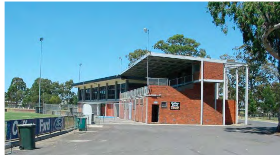
Shepley Oval Pavilion. This pavilion is an important sport and cultural facility. Any improvements and extensions will require universal access and should also interact positively with the parklands and not create an unfriendly southern side to the parklands and Creek.
