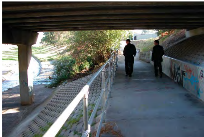
Existing McCrae Street bridge underpass
