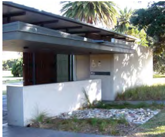
Indicative toilet block (Centennial Park, Sydney). Rough concrete walls, shared washing zone and timber screens.
