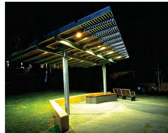
Indicative shelter block. Tall metal structure with timber panelling for shade and low concrete walls as seating and edge treatment.
