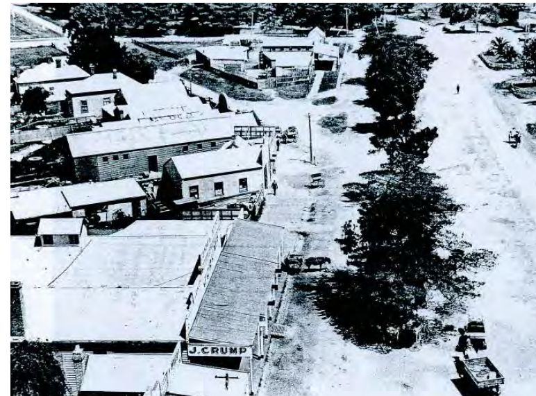
Elevated view of Dandenong looking along Lonsdale Street towards Dandenong Park in early 1900s.
