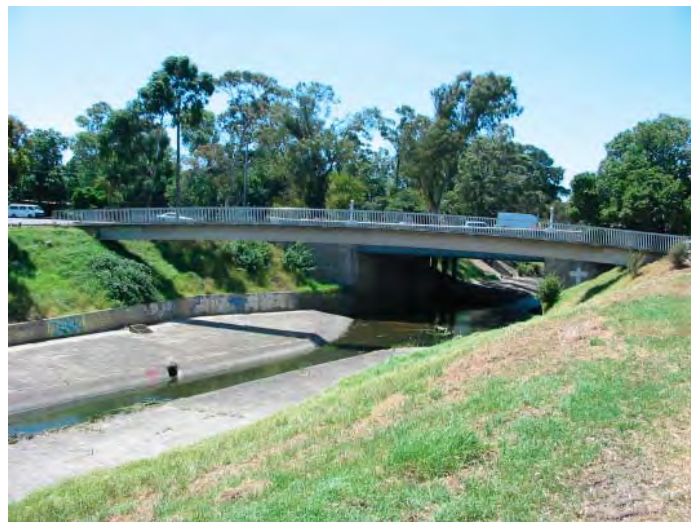
Potential underpass - Princes Highway
