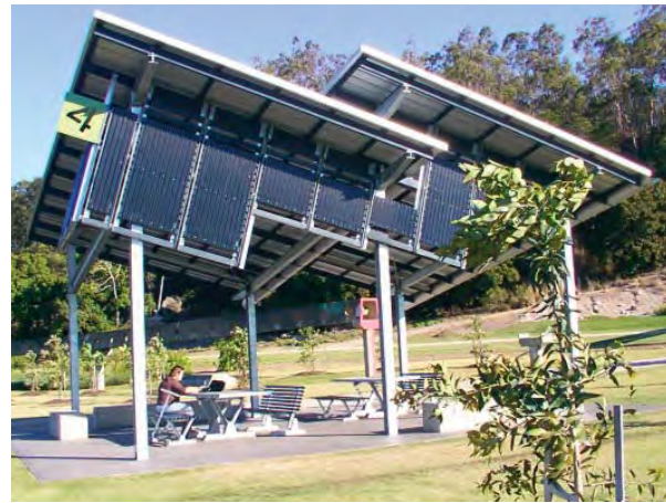
Indicative shelter block (Rocks Park, Brisbane). Tall metal structure, solar panels and low concrete walls as seating and edge treatment.
