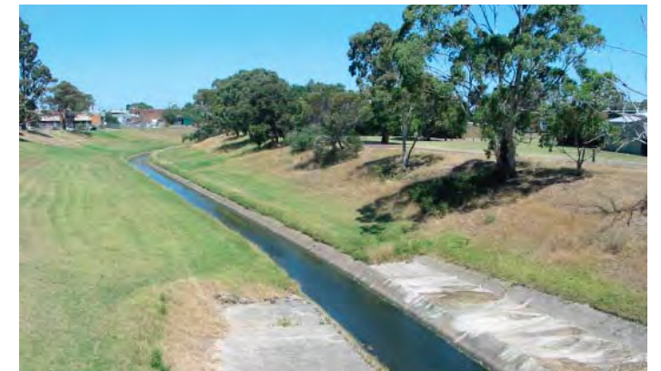
Existing conditions of Dandenong Creek with concrete channel.
