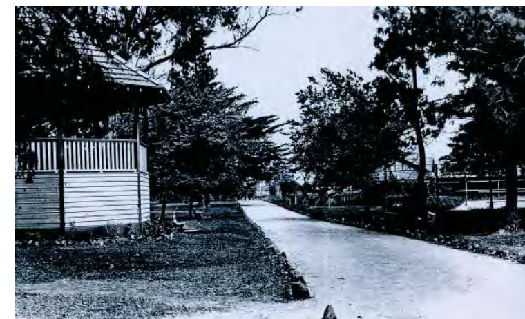
Historic wooden bandstand.
