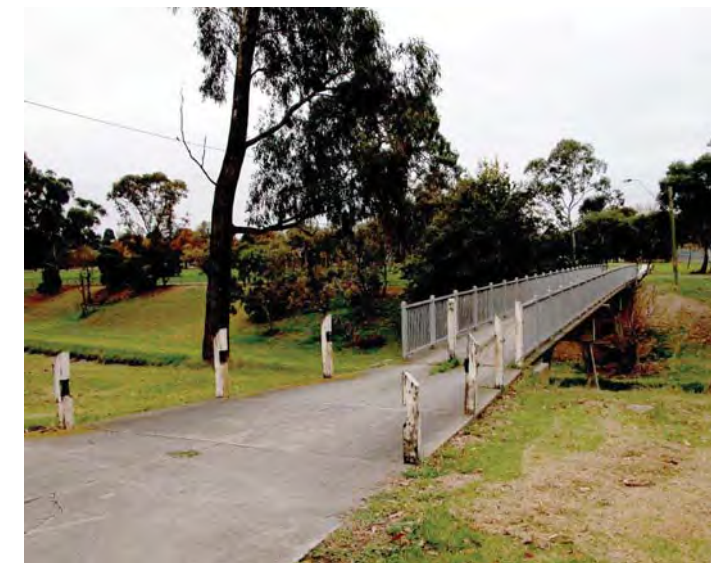
Existing Pedestrian Bridge over Dandenong Creek.
