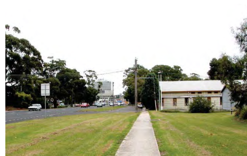
Old Army Drill Hall
