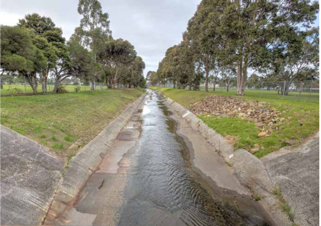
Mile Creek downstream Springvale Road – concrete-lined channel
