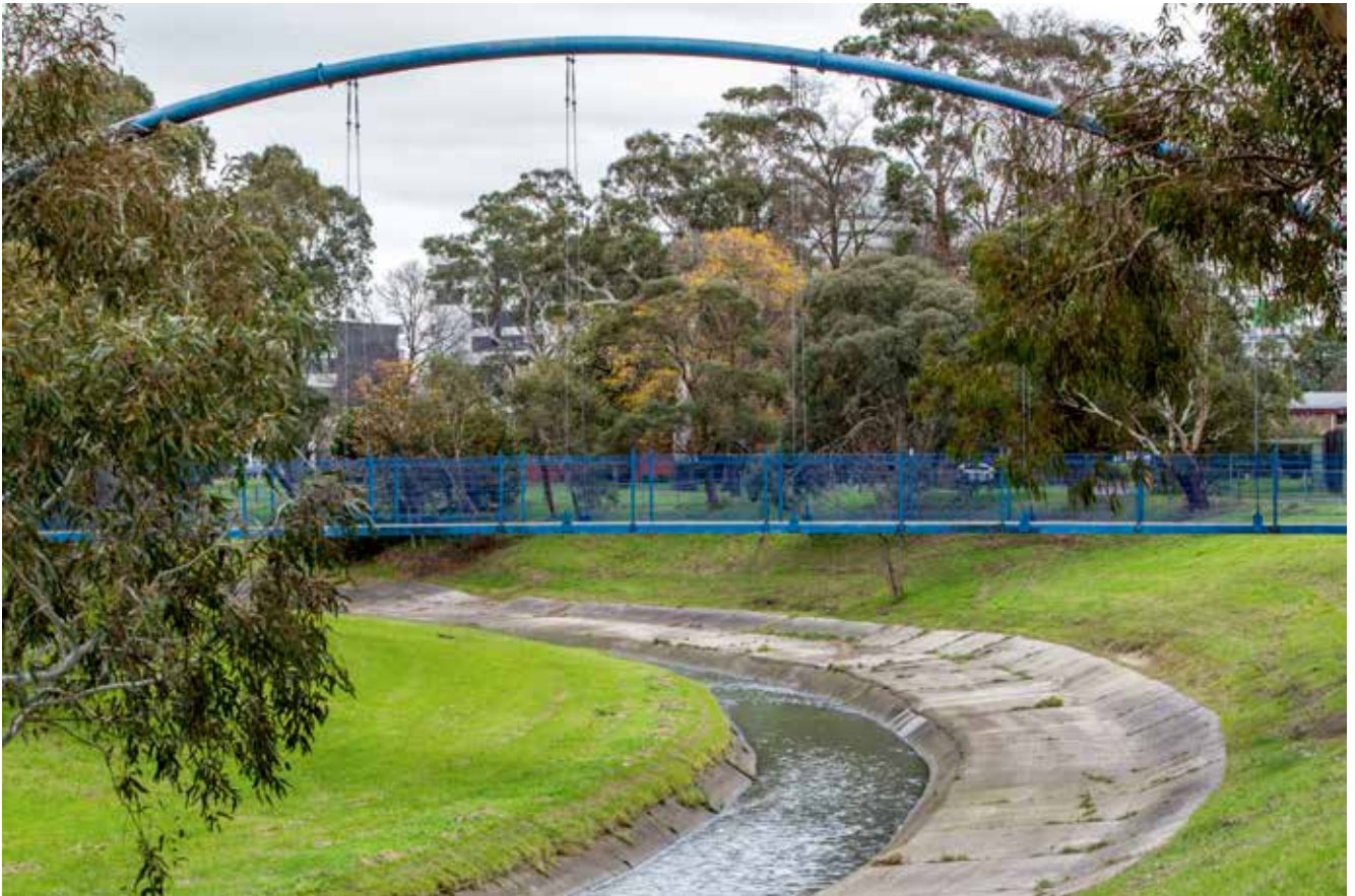
Dandenong Creek downstream Lonsdale St – concrete-lined channel
