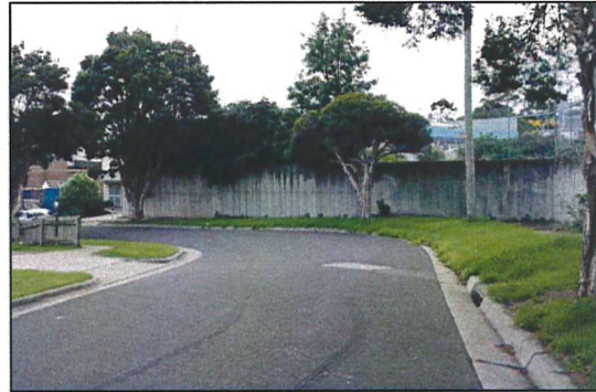
Photo 6 Retaining wall along Carmen Street frontage
