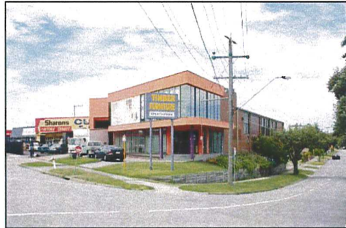
Photo 2 Two storey industrial building 223 Princes Highway
