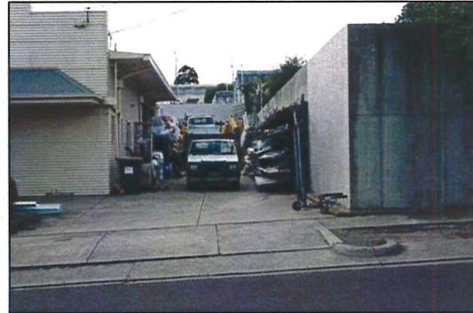
Photo 8 Entrance to Access Roofing showing retaining wall along boundary of subject land
