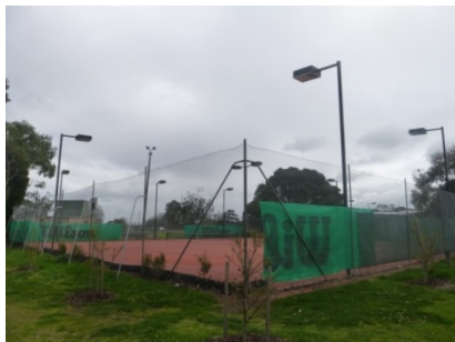
Existing Tennis Courts
