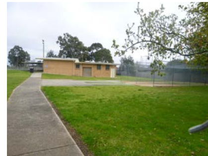
Existing Parkfield Pavilion
