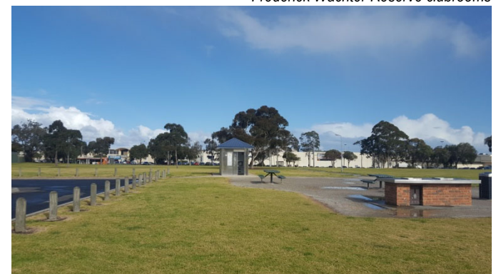
Public Toilet south
