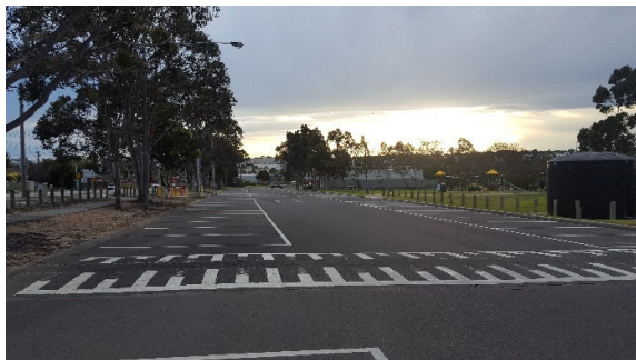
Main car park
