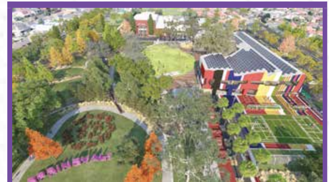
Springvale Library will be constructed to achieve a 5-star Green Star rating and be Council's first zero net emissions building.
