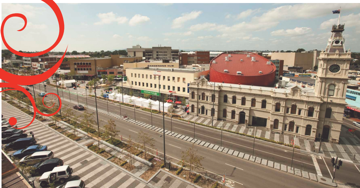
$20 million transformation of Lonsdale Street, Dandenong has been completed.
