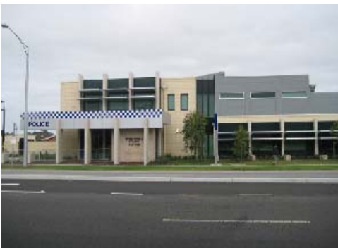
The new Police Station located at part of Eriksen Garden
