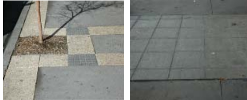
Flagstone Paving with In-situ Concrete or asphalt Infill. Adopt for secondary streets such as Balmoral, Windsor and Saint James Ave
