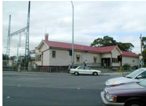
The Springvale Station building sits alongside busy Springvale Rd
