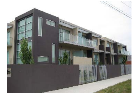
Cnr of St James and Buckingham Ave. Sixteen apartments under construction with basement car parking on a lot size of 1210 m2. A significant first step in higher density residential living in Springvale
