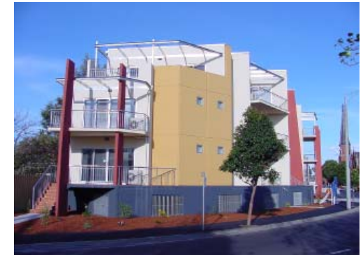
Basement parking should be encouraged to maximise the potential of the site area and contribute positively to the building form
