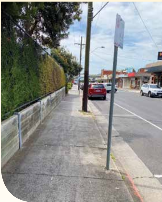
Bottom left. Planting opportunities in Buckley St, which would require a designed planting response
