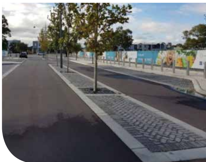
Figure 6. Permeable pavement incorporated into linear planting vault Nuytsia Way, Brabham, Western Australia (New Water Ways, seen at newwaterways.org.au/projects/nuytsia-way-brabham )
