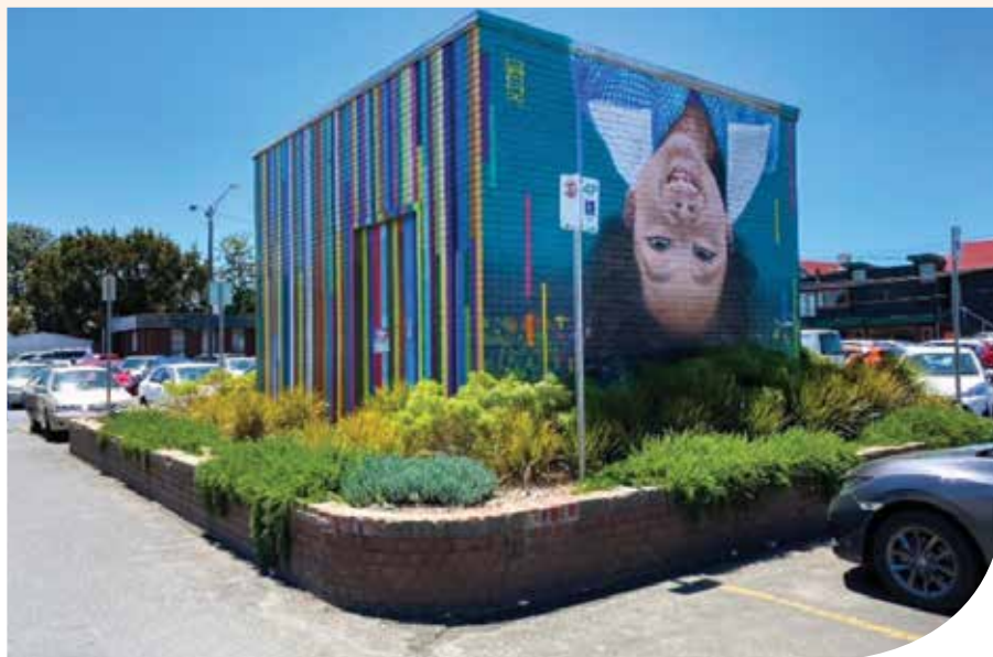
Substation in Warwick Avenue car park north.
