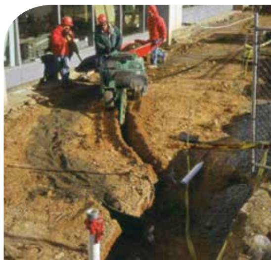
Figure 4. Excavating tree root channels during pavement reconstruction works
