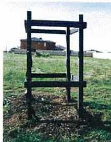
Tree Guards Painted Timber
