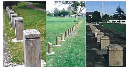
Timber Bollards Cypress Pine Timber
