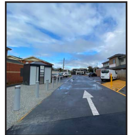
HEMMINGS STREET CARPARK UPGRADE (COMPLETED 2021)
