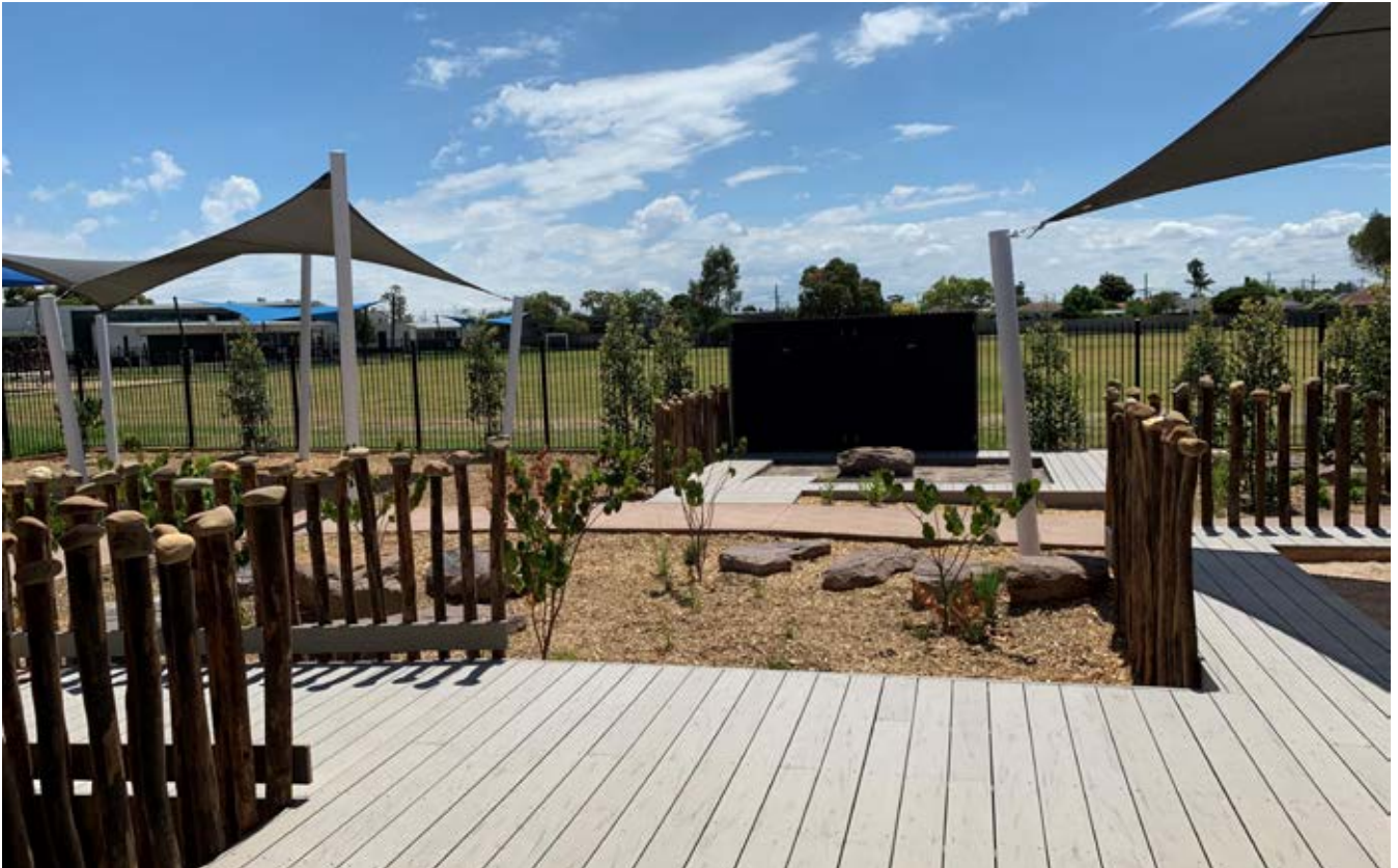
Keysborough Primary School Kindergarten
